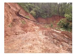
Fig. 2. Slope failure in cut slope
